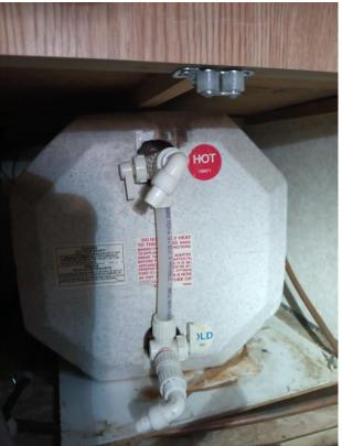
Remove the tank by pulling it from outside the coach. If it's too difficult, break away the Styrofoam from the HW tank for easier removal.
