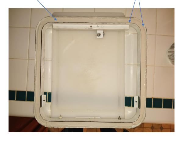
Put the frame in place and add the 3 cover screws.
