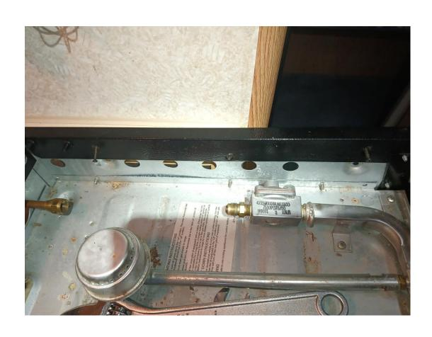
Turn on the propane and test for leaks using soapy water near the threads or better yet put your nose right to the fitting and smell. If gas is detected then more than likely the fitting requires tightening. If no gas is detected continue on.
