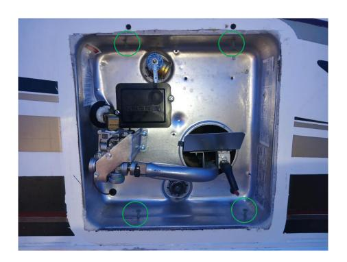
Add the <u>Butyl</u> tape to the perimeter of the frame and a bead of silicone, along <u>each</u> side of the Butyl
